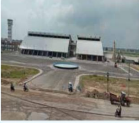
View of Control tower and ITB
